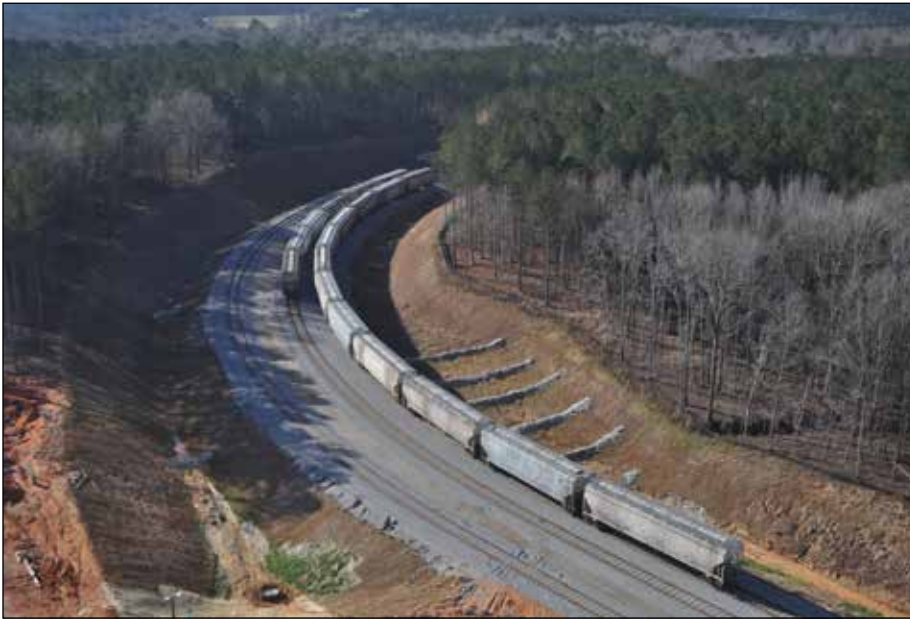
8,200-foot loop track off the CSX railroad has a 125-car capacity.
